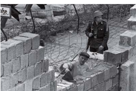
The Berlin Wall was first made of brick and barbed wire, but was later erected in cement and steel.
